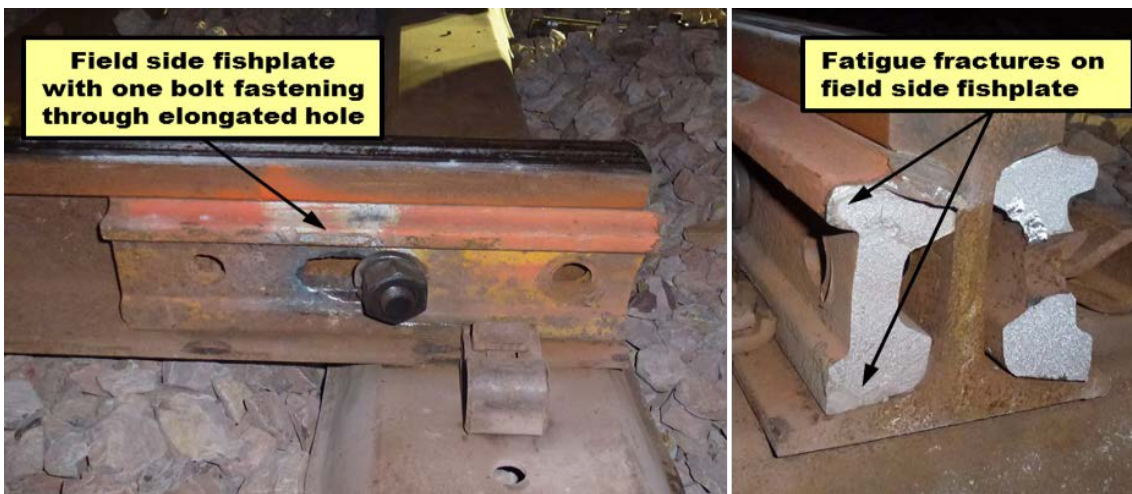
Figure 5: Southern rail joint
